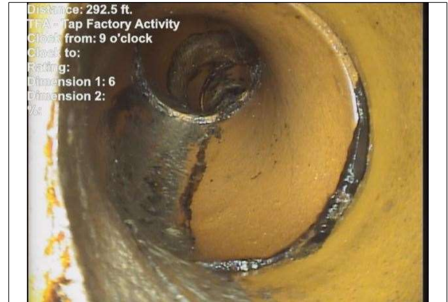
At: 292.5 ft. 9/. TFA - Tap Factory Activity Joint: No
