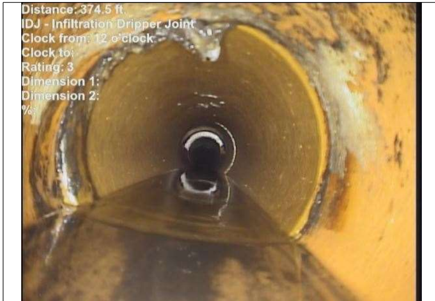
At: 374.5 ft. 12/. IDJ - Infiltration Dripper Joint Joint: Yes
