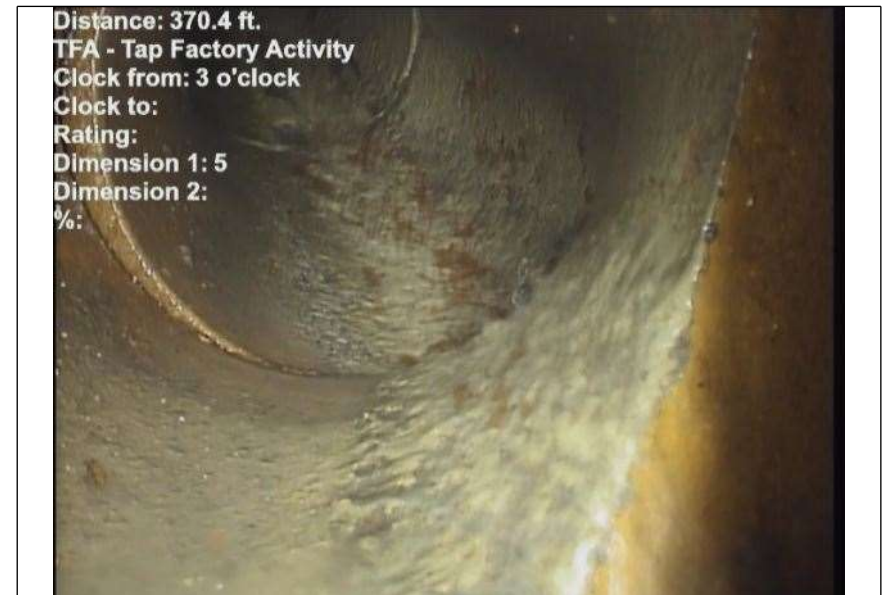
At: 370.4 ft. 3/. TFA - Tap Factory Activity Joint: No
