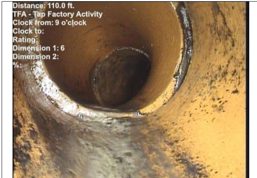
At: 110 ft. 9/. TFA - Tap Factory Activity Joint: No
