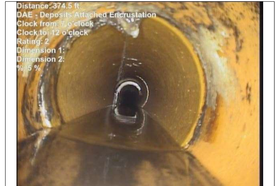
At: 374.5 ft. DAE - Deposits Attached Encrustation 7/12 Joint: No 5 %
