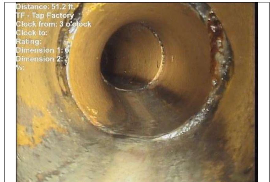
At: 51.2 ft. 3/. TF - Tap Factory Joint: No
