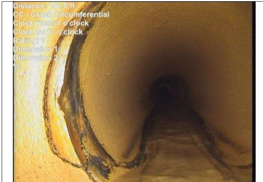
At: 144.8 ft. CC - Crack Circumferential 8/11
