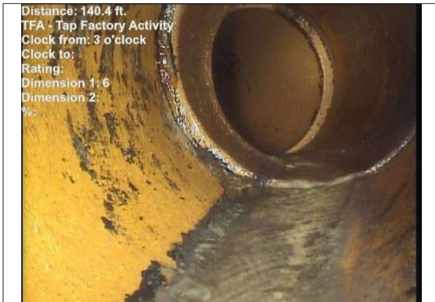
At: 140.4 ft. 3/. TFA - Tap Factory Activity Joint: No
