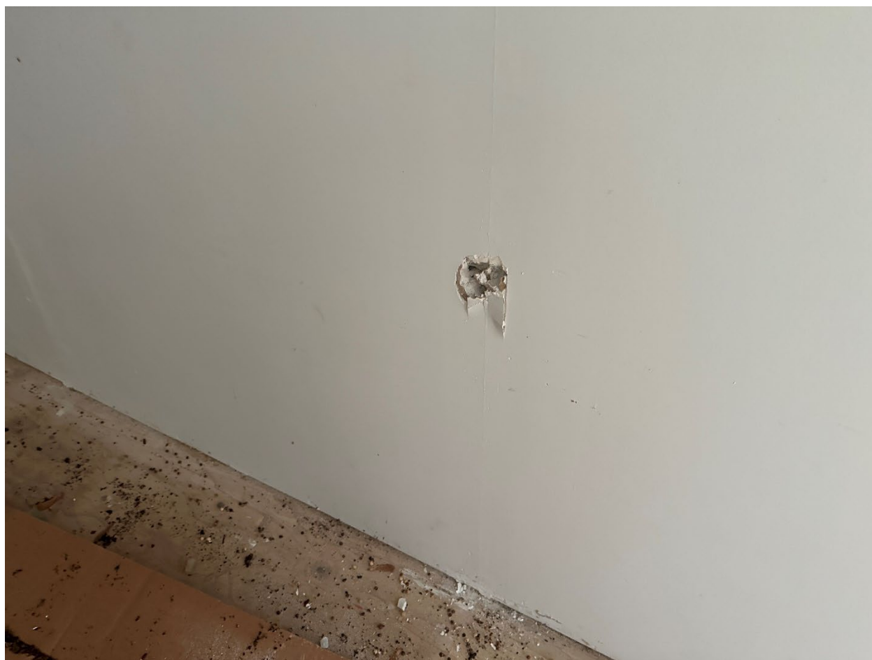
Photo 3 – View of the drywall (wall) in the loft where 03-A was collected.
