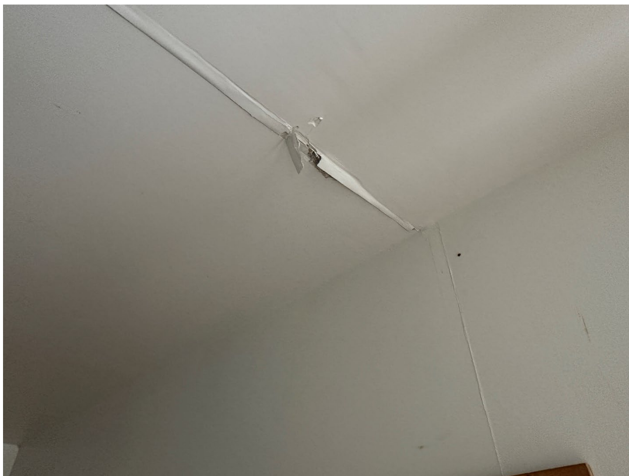
Photo 2 – View of the drywall (ceiling) in the loft where 04-A was collected.
