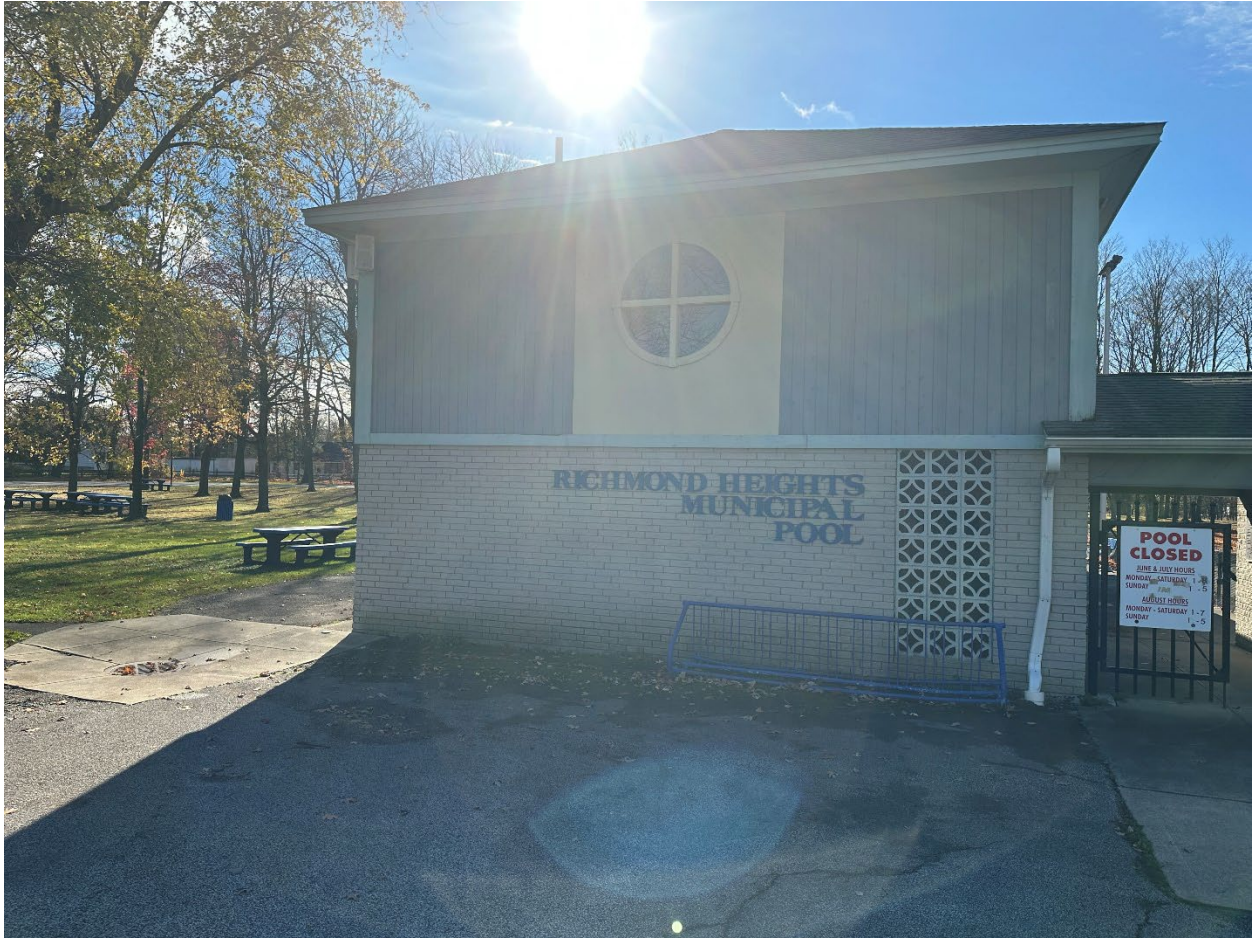
Photo 1 – Photo of the northern side of the L-shaped building where all asbestos samples were taken.
