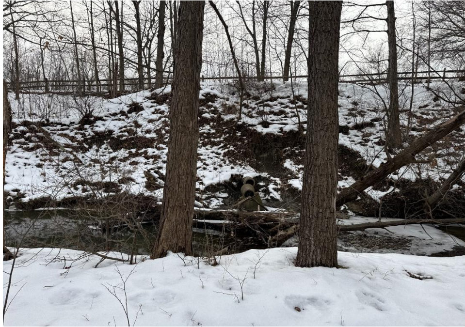
Photo 7: This photo shows a closeup from the east bank of the creek, looking north, highlighting the slope condition on the west bank. A broken drainpipe is visible at the bottom of the slope.
