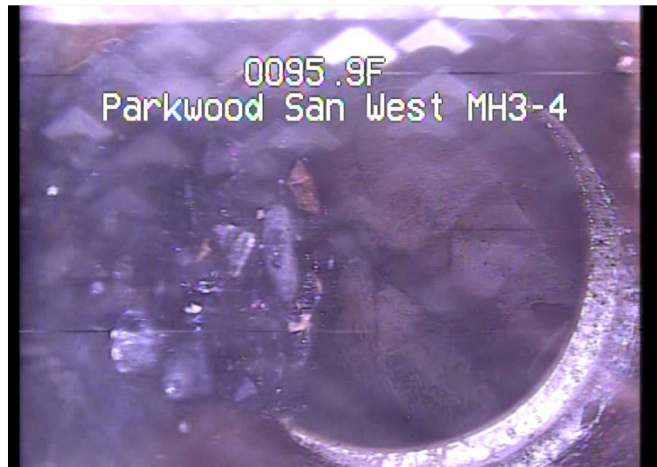
Photo 2. Lateral Point Repair
